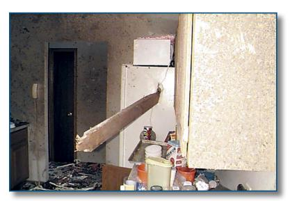
2" x 6" missile penetrating a refrigerator, Midwest Tornadoes of May 3, 1999 doors in a building should be opened to equalize the pressure. In fact, opening a window or door allows wind to enter a building and increases the risk of building failure.
